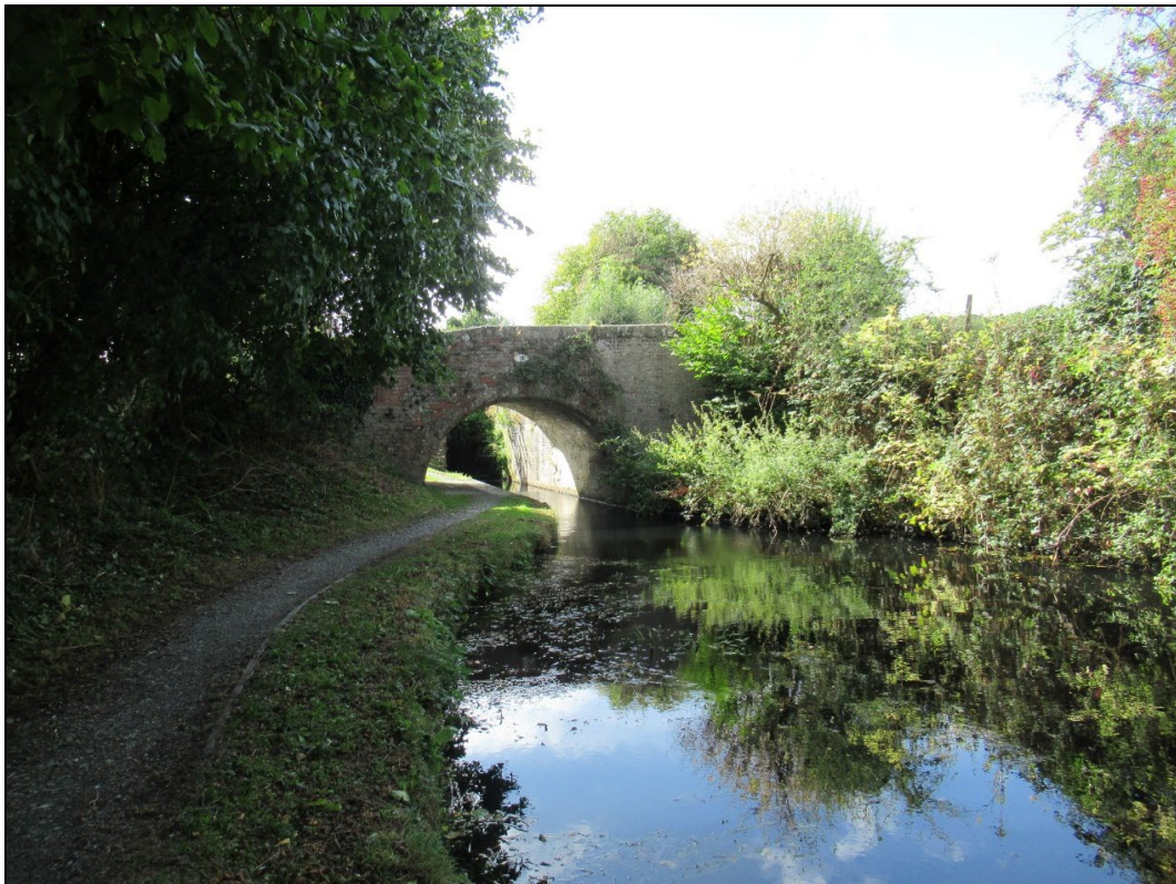
Plate 6: PQY2025_006. Bridge 111, Listed Building 16773, seen from the towpath to the north-northeast of the bridge. Looking south-southwest.
