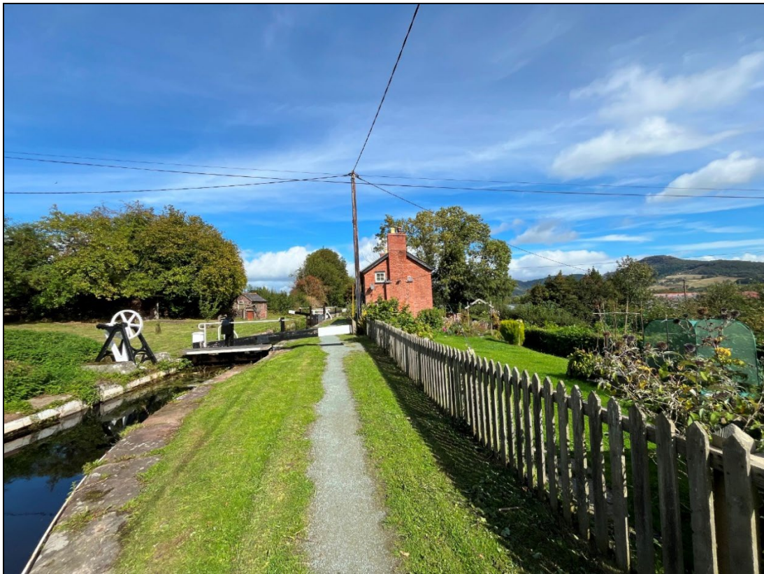
Plate 16: PQY2025_016. A view of Top Lock, to the left, with Lock Cottage to its right. Looking north-northeast.
