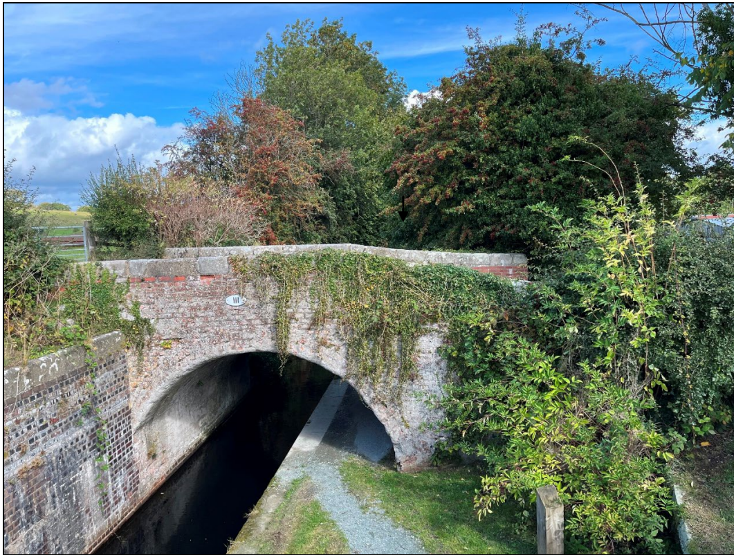
Plate 5: PQY2025_005. Bridge 111, Listed Building 16773, viewed from Top Lock, Listed Building 16772. Looking north-northeast.
