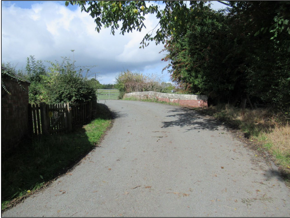
Plate 9: PQY2025_009. A view towards the top of Bridge 111. Looking north-northwest
