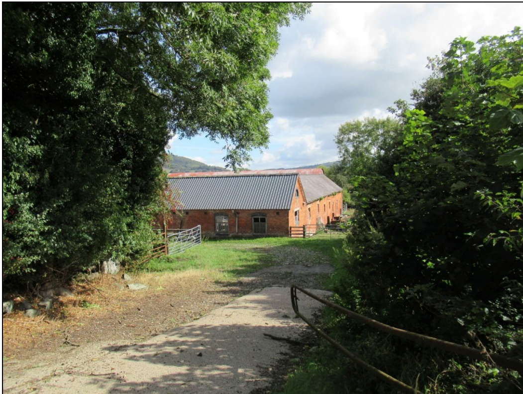
Plate 23: PQY2025_023. A view of the brick farm buildings at Bank Farm, seen from the minor road just to the southeast of Bridge 111.
