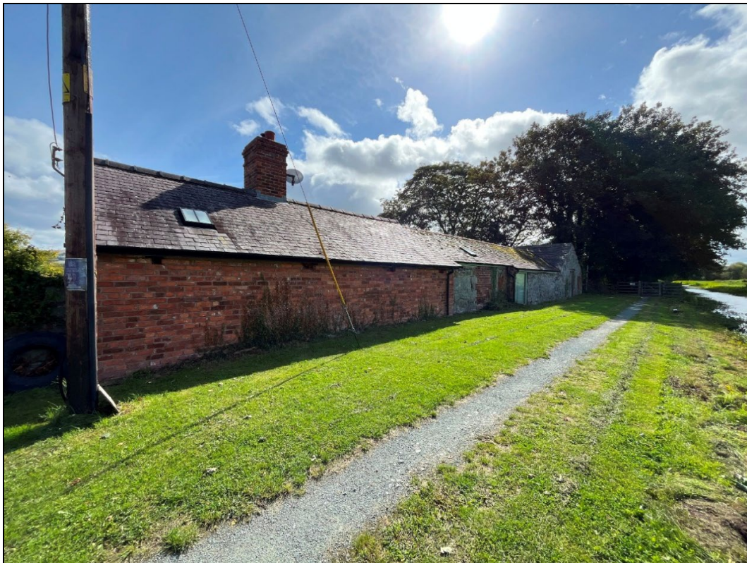
Plate 12: PQY2025_012. A view of Ivy House and its outbuilding which was formerly a warehouse on the canal side, and prior to that part of a largely lost complex of industrial buildings. Looking south.
