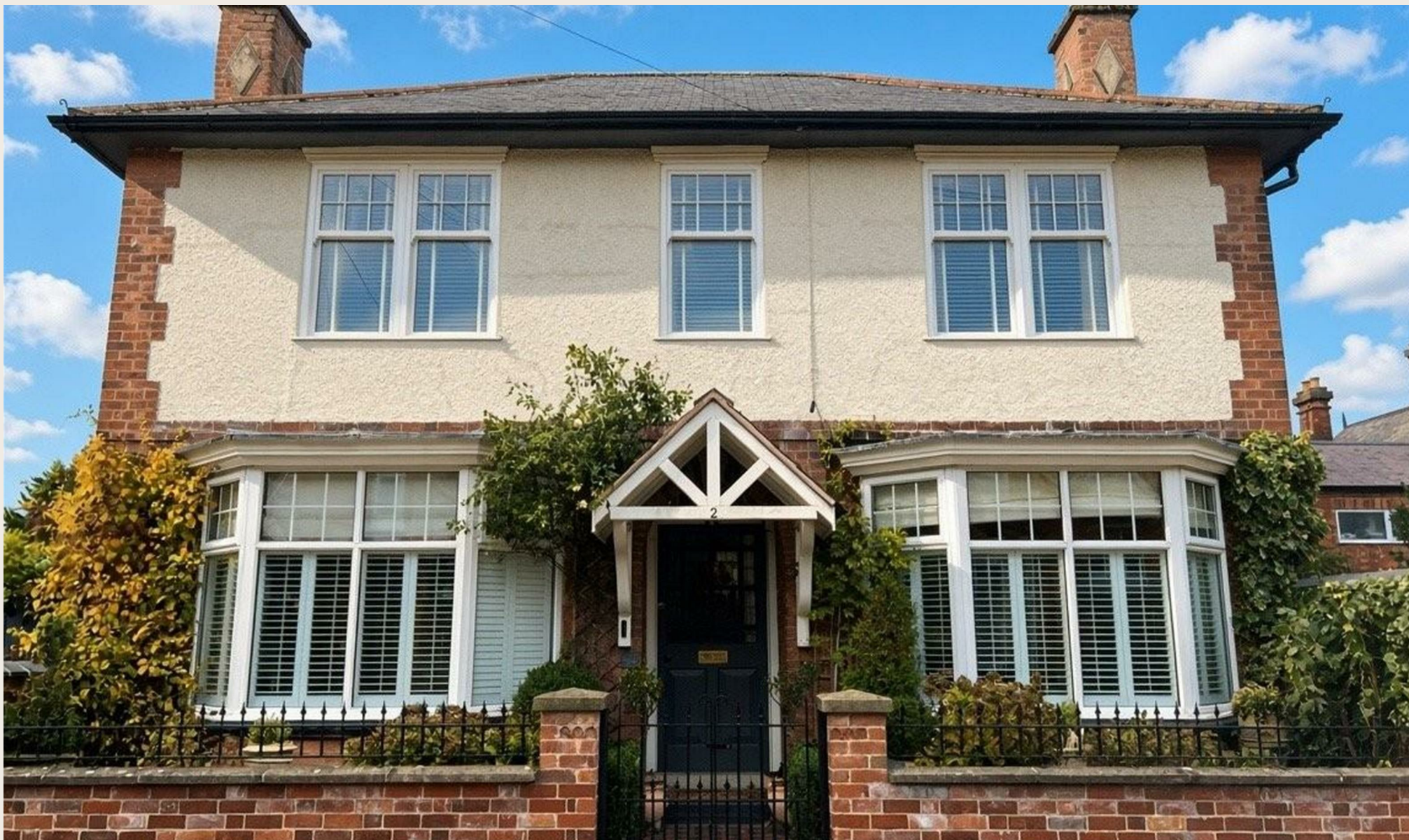
Alken House, 2 Cottessmore Avenue, Melton Mowbray, LE13 OHY £435,000
