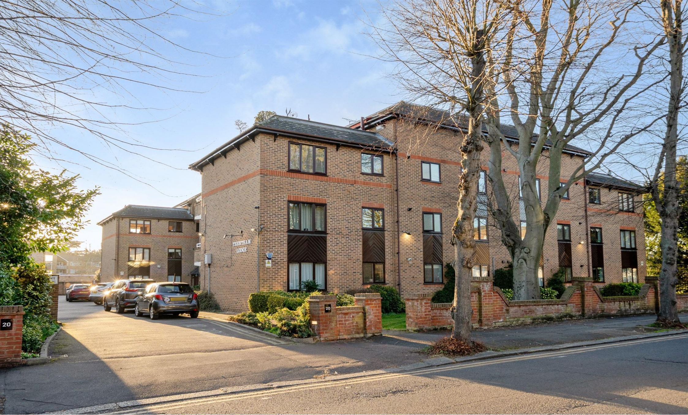
Trentham Lodge, Wellington Road, Enfield, EN1 2PD
