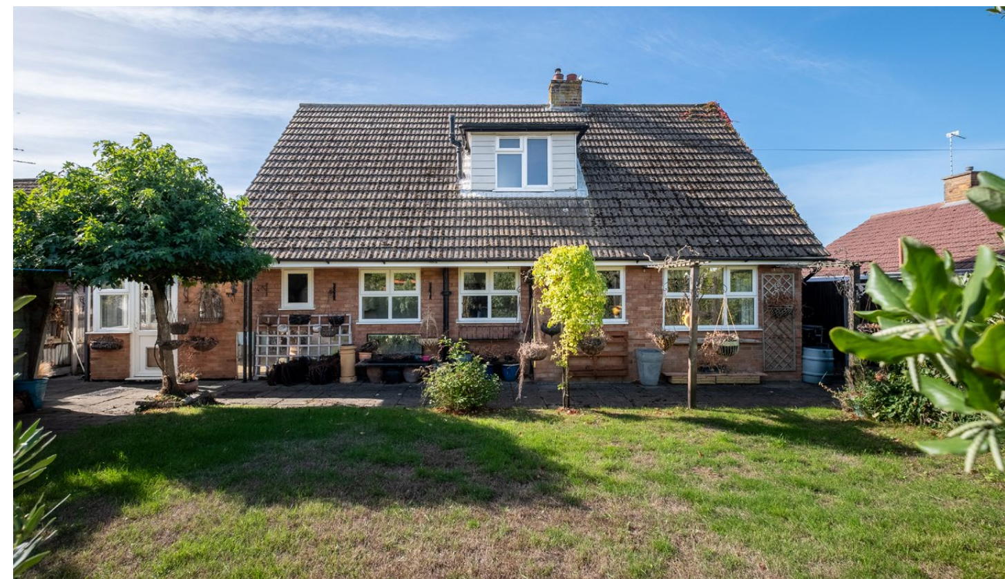
The rear facade
