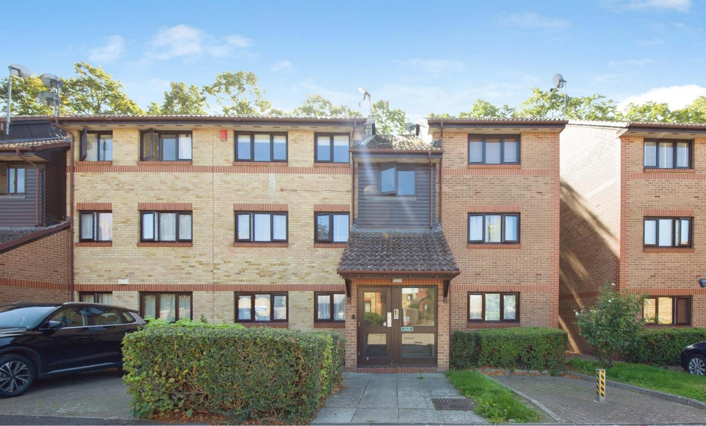
Waterside Close, Barking, IG11 9EN
