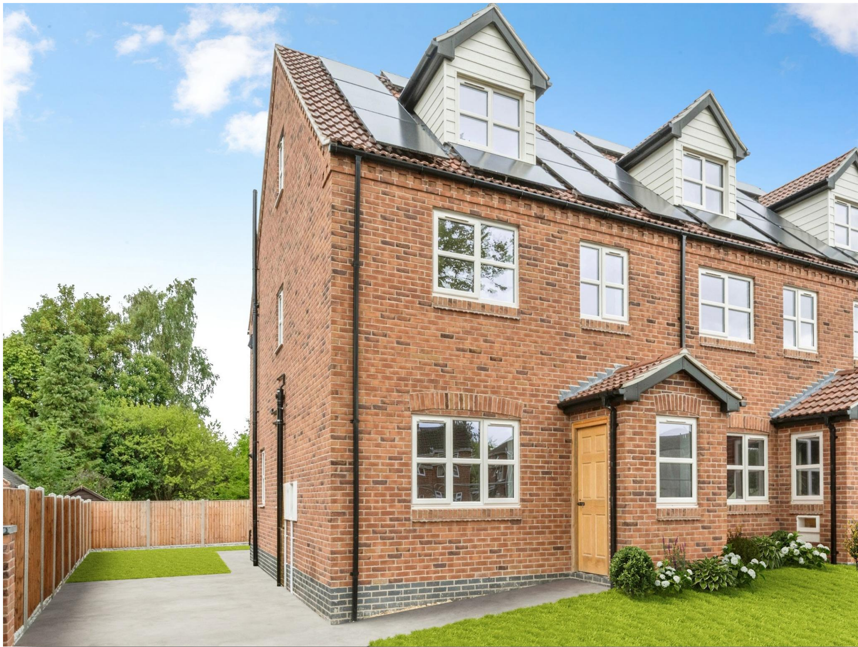
Unit 2 West Street, West Butterwic DN17 3LA
