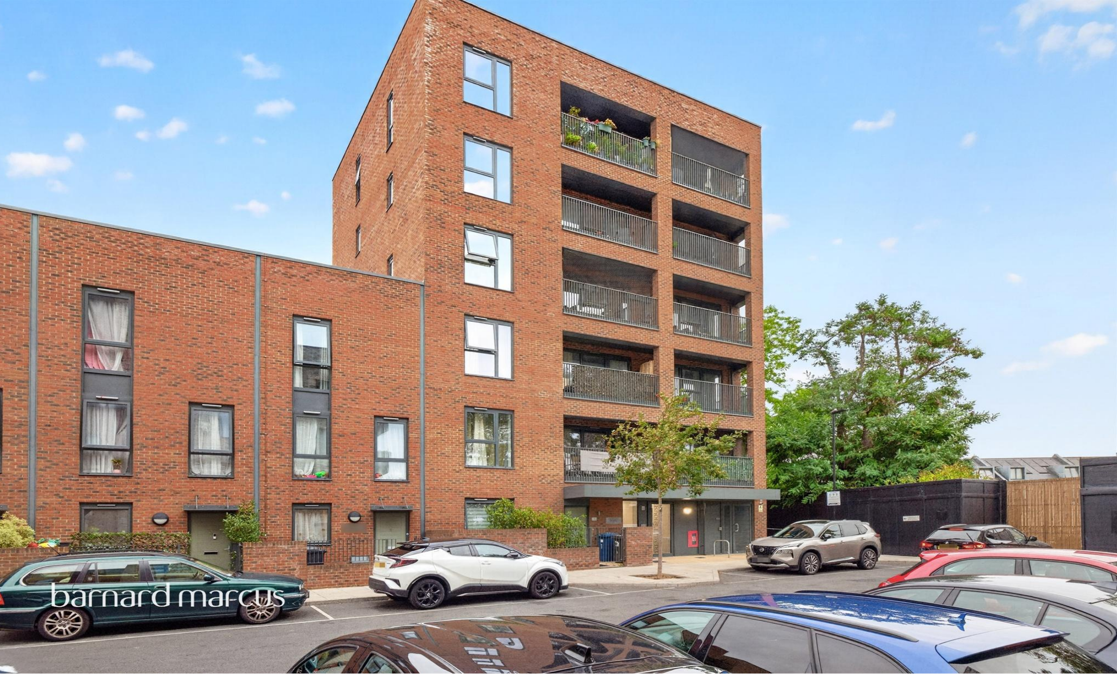
Tremlett Building, Tewkesbury Road, London, W13 0FS
