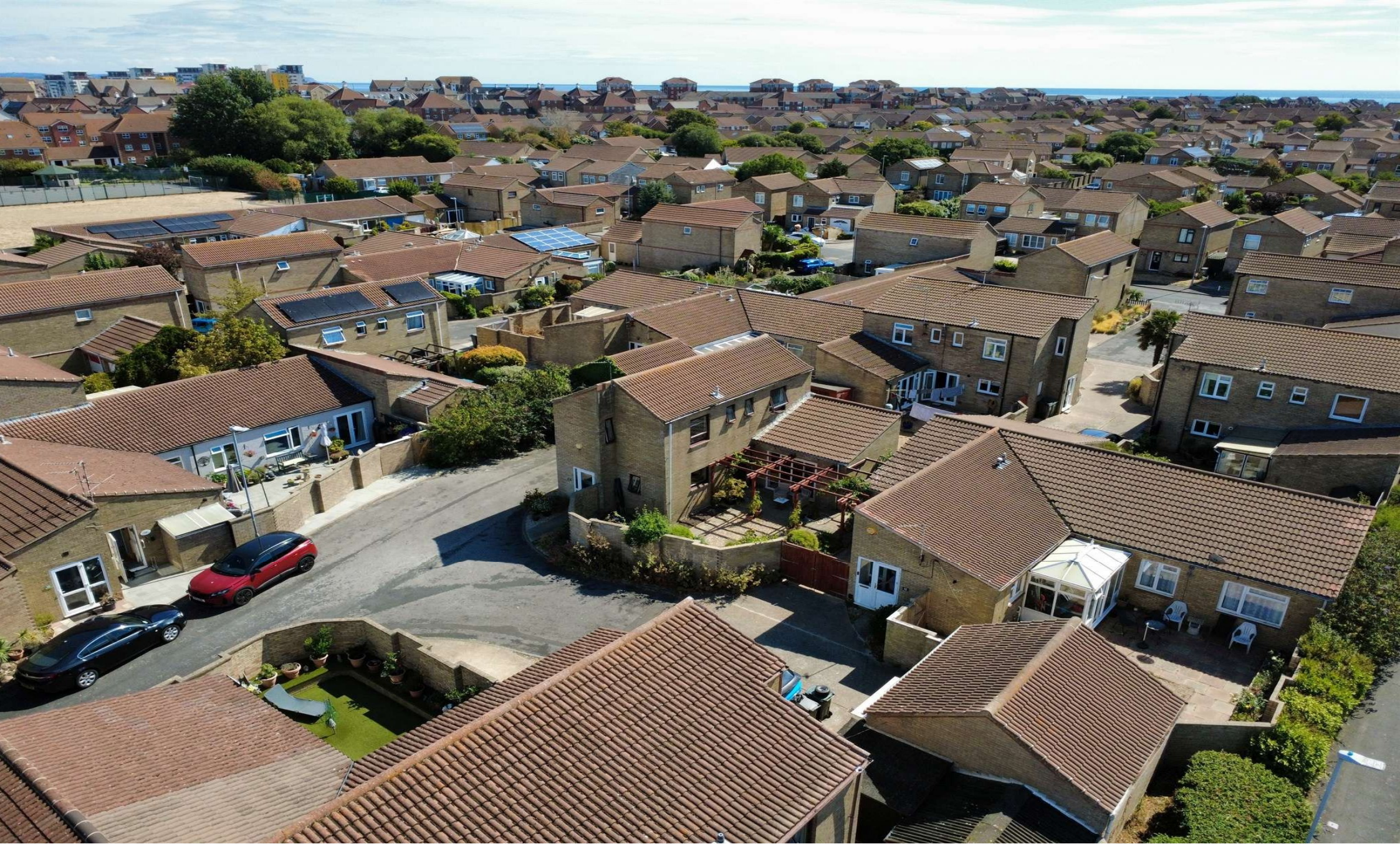
Gardner Close, Eastbourne BN23 6DQ
