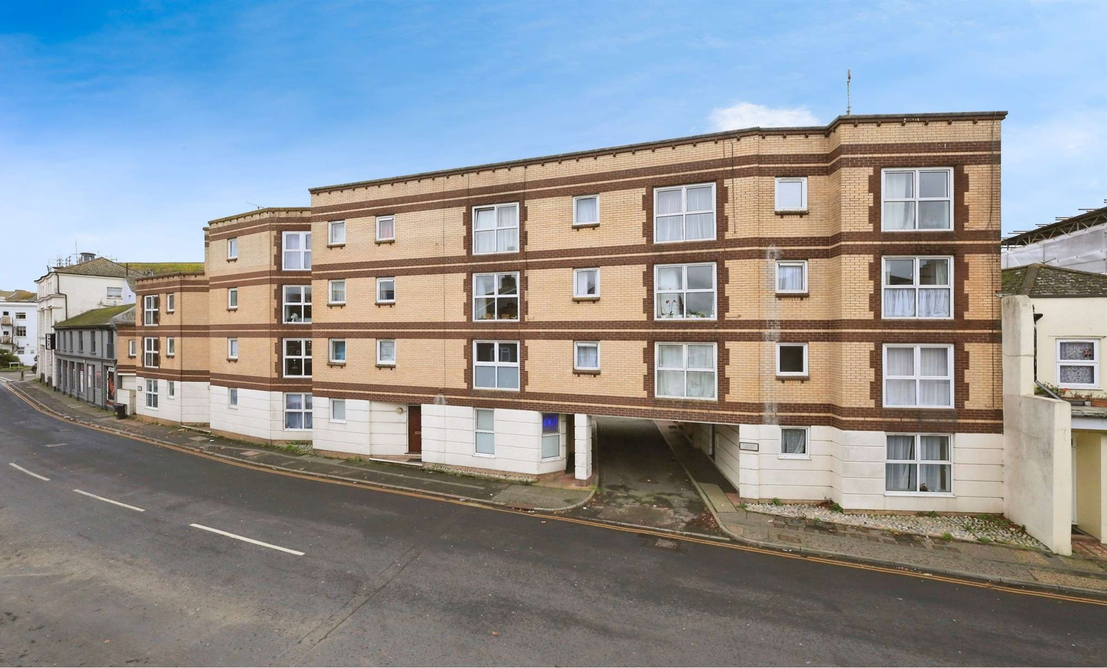
Phoenix Court Langney Road, Eastbourne BN22 8AJ
