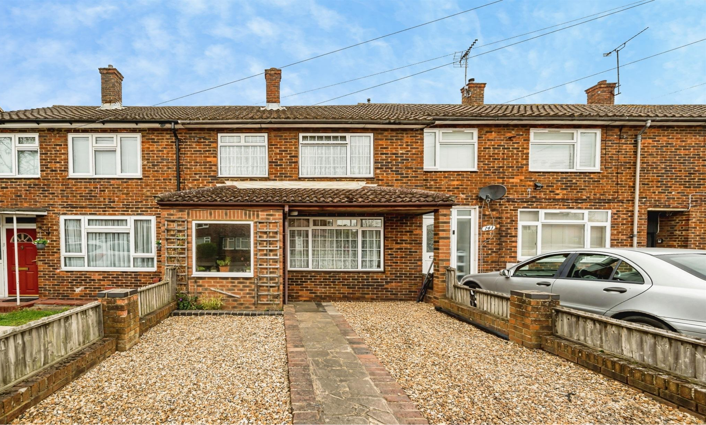
Long Readings Lane, Slough SL2 1QY
