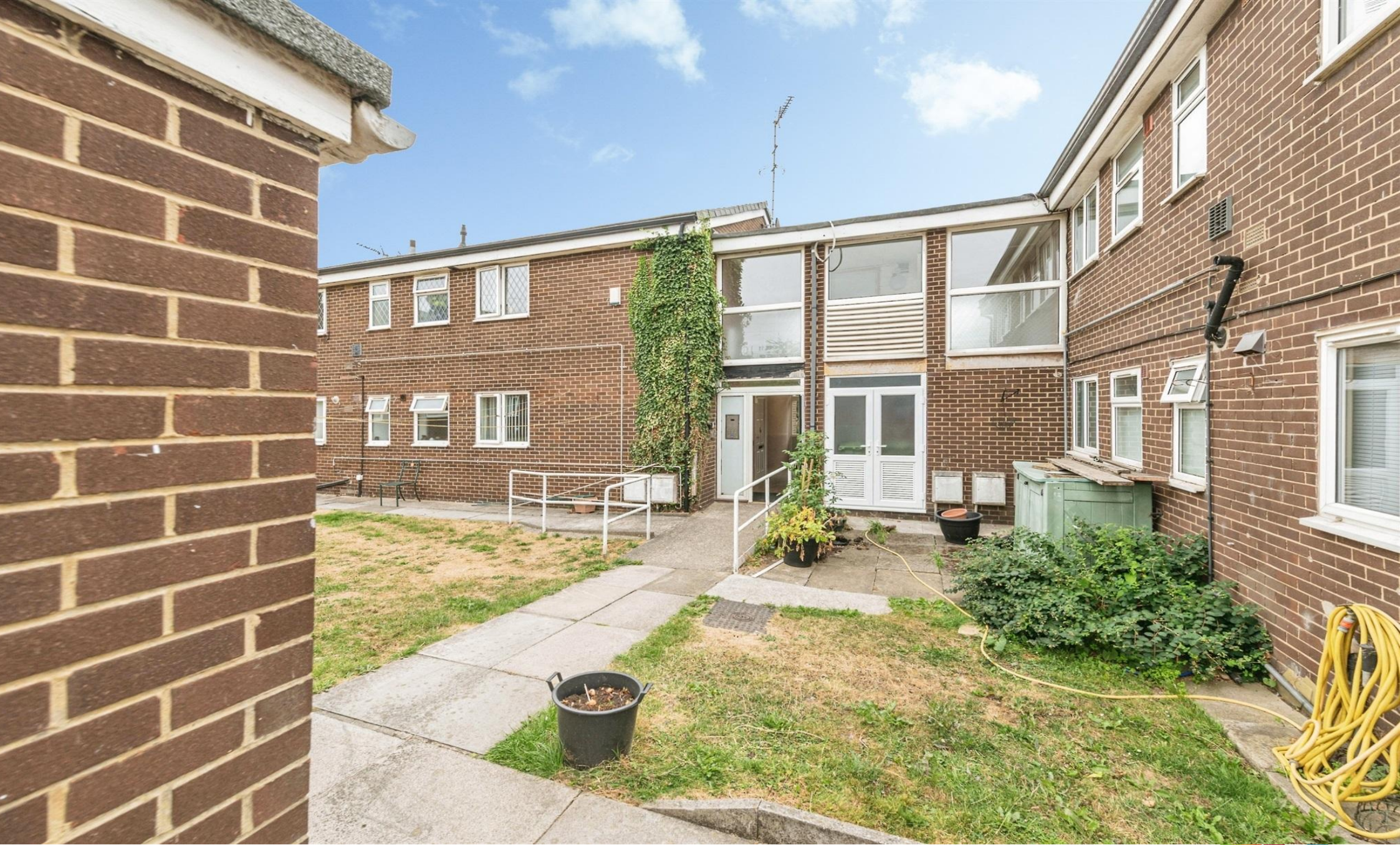
Bridge Close, Horbury WAKEFIELD WF4 5QB
