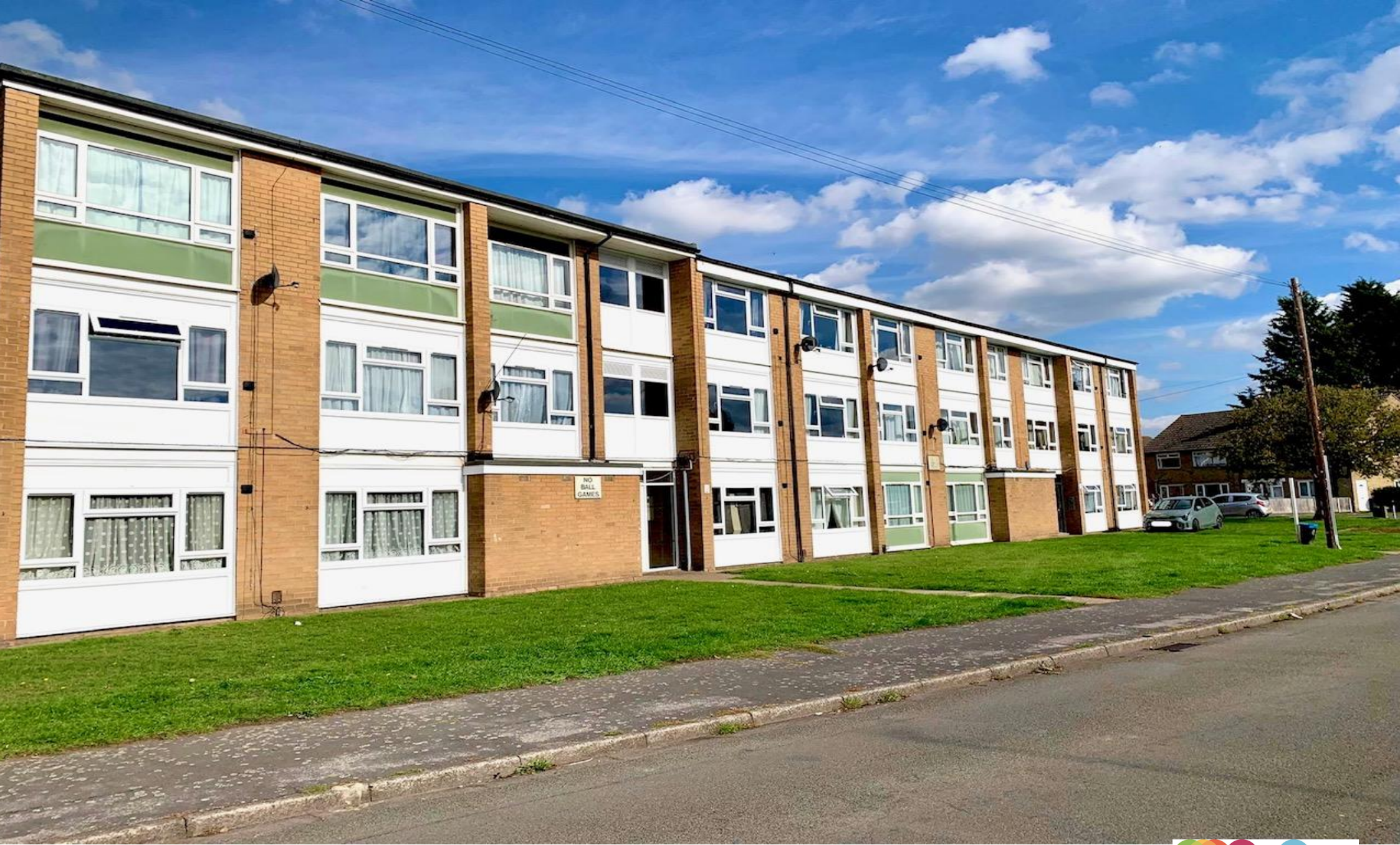
Camwood Crescent, LINCOLN LN6 0PH
