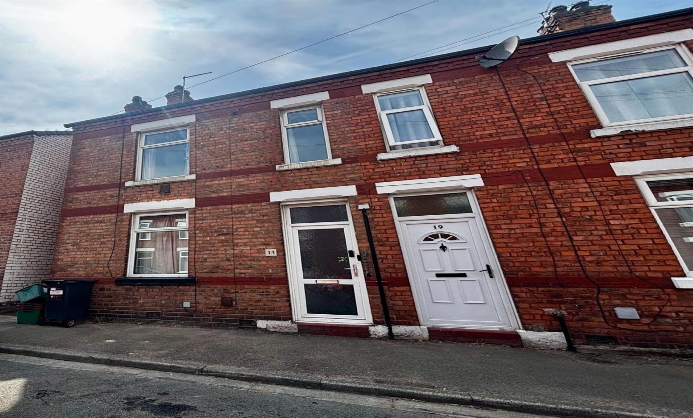
Bond Street, Northwich CW8 4DG
