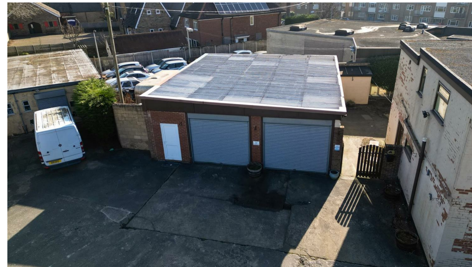
Rear Workshop, Littlemoor Service Station, Chesterfield
