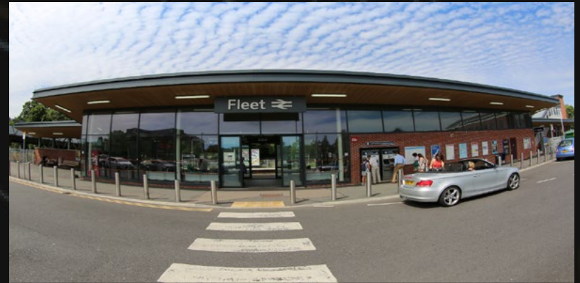
Fleet Mainline Railway Station
