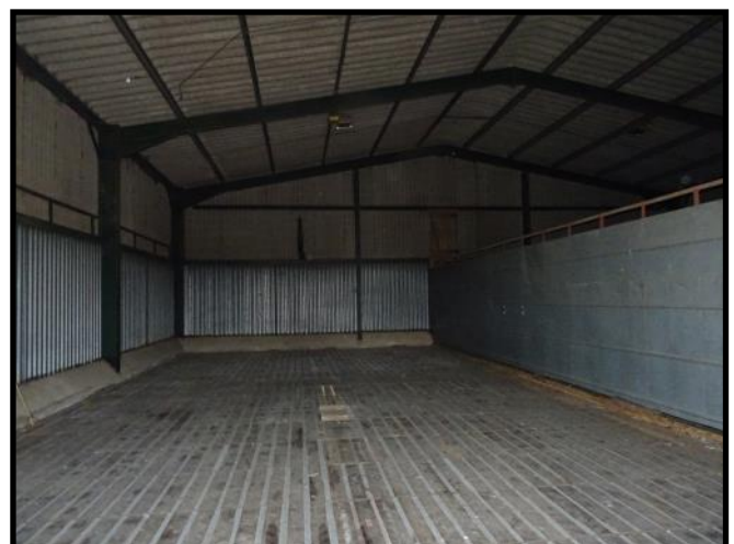
Internal view of grain storage (Northern building -eastern side)
